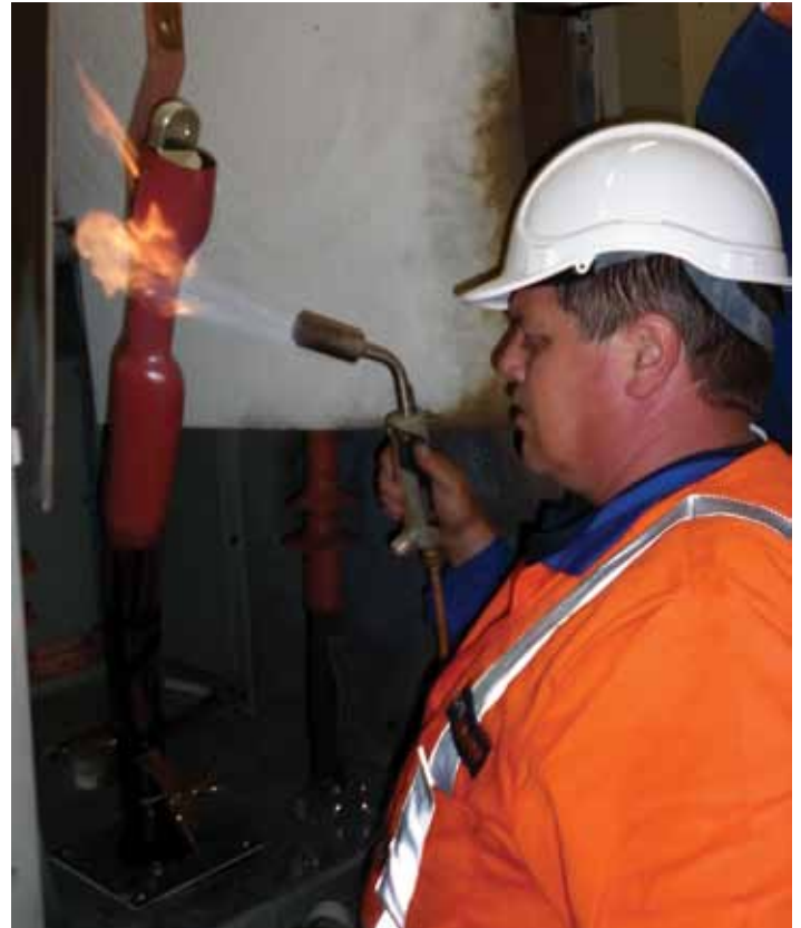
Rob Dickerson assists on a 33kV fault
