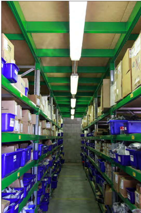
Before: Low level picking aisle illuminated by fluorescent tubes, poor light spread.
