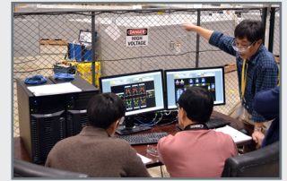
System Automation and Smart Grid Solutions
