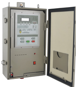
◀ Automated controller with FTU-P200C
