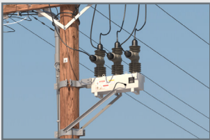
Three Phase Overhead Load Break Switches
