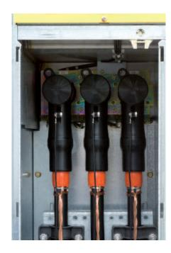
Raychem screened separable connectors RSTI-58 are designed to connect single- and three-core polymeric cables to medium-voltage gasinsulated switchgear and other equipment using CENELEC bushings type "C" specified for 630/1250 A up to 24 kV. Made of
