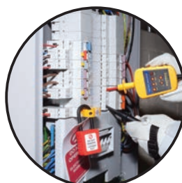
Test the supply is isolated.
