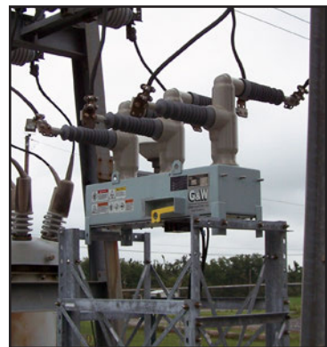
▲ Custom mounted frame required for replacement of previously installed oil filled equipment.
