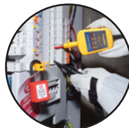
Test the supply is isolated.
