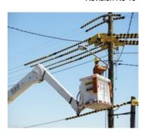
The **Balmoral™** Lion Tails™ (Line Guards) are designed to cover Power Lines and Wires to provide electrical insulation from brush contact and mechanical protection. Additionally they give a distinct visual warning around building and construction sites and importantly where live works and maintenance is being carried out.
