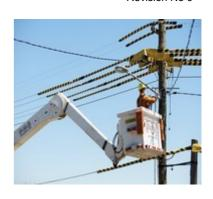
The **Balmoral™** Tiger Tails™ (Line Guards) are designed to cover Power Lines and Wires to provide electrical insulation from brush contact and mechanical protection. Additionally they give a distinct visual warning around building and construction sites and importantly where live works and maintenance is being carried out.
