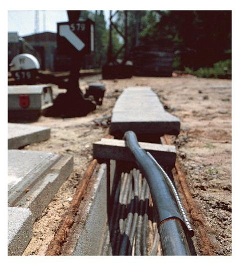
CRSM wraparounds are used in a railway goods yard in Germany to restore the insulating, sealing and mechanical protection functions of damaged cable oversheaths.
