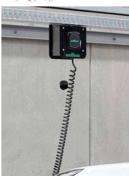
This is the perfect solution for body corporates or building owners to make the building EV ready. All that is required is a DB9 switchboard, cable tray and a power sharing junction box - then it's up to the individual carpark owners to take advantage by adding a Wallbox charge station.
