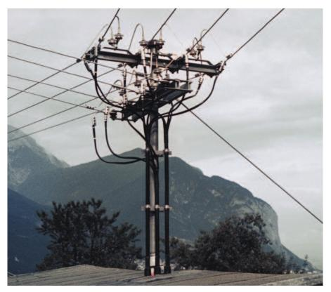
An electrical system in Austria. Raychem tubing MWTM protects and seals the cable cores and connectors as part of a Raychem termination, and seals the cable feedthrough into a building.
