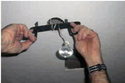
1. Attach light into bar.
