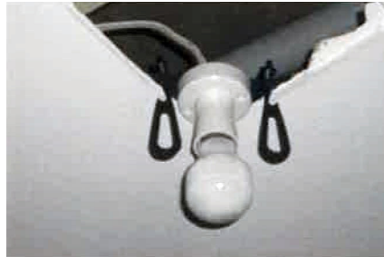
5. Secured to ceiling.
