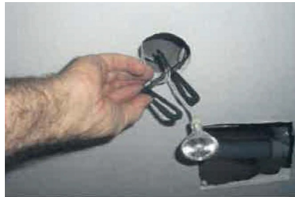
2. Insert into ceiling cavity.
